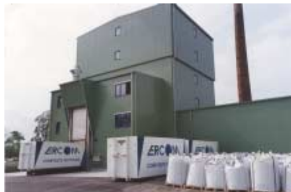
The Ercom recycling plant at Rastatt
